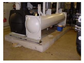
Air Springs with rubber-to-metal-bonded structure
